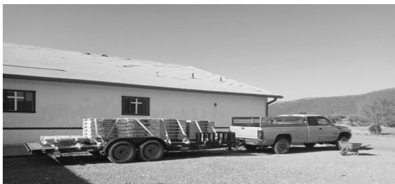
New roofing will be put on soon.
